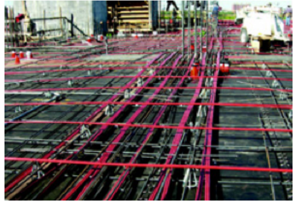
Figure 12: Post-Tension Tendons
